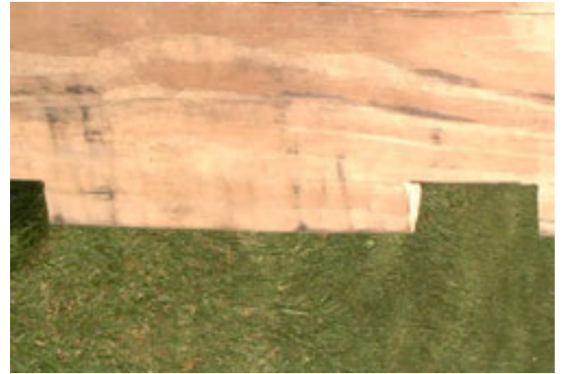
Notch the arbor rafters for a tighter fit.
