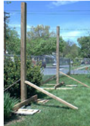
Ensuring the posts remain plumb by bracing them with scrap lumber. David Beaulieu
